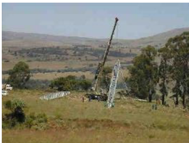
Raising the pylon
