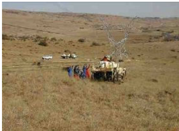
Stringing pilot cable with pilot tractor
