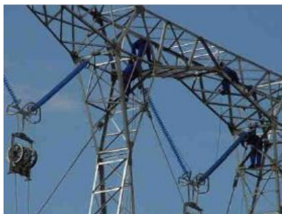
Using pulleys to hoist cable
