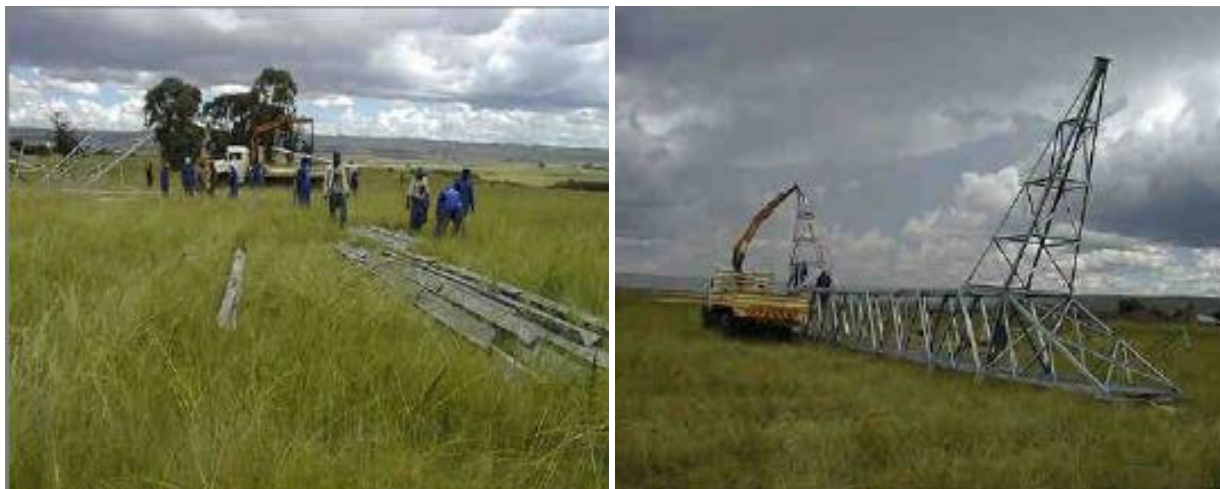
Steel delivered for assembly
